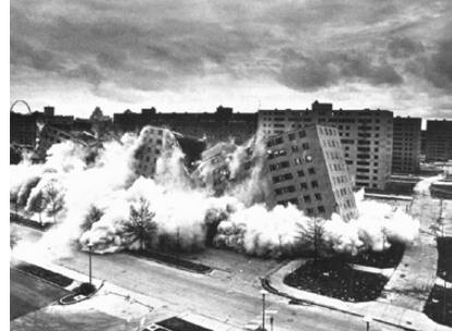
Demolition Minoru Yamasaki's Pruitt-Igoe housing project, St Louis, July 15 1972
